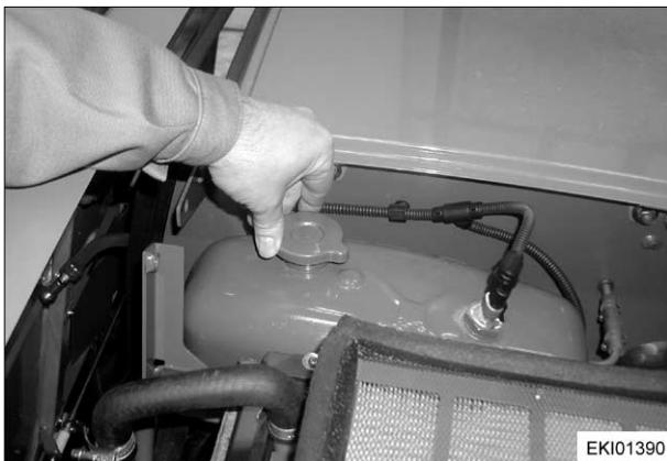
Carefully open coolant-water cap.
