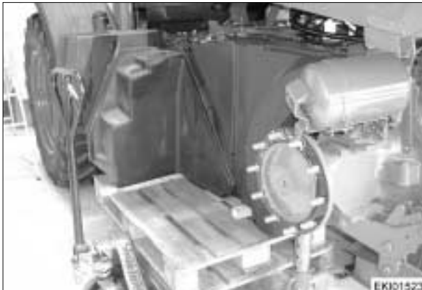
Fitting fuel tank and auxiliary tank
