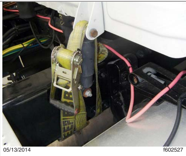
Fig. 24.8, Tension Strap Installed to Hold Down the Cab
