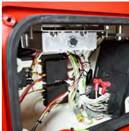
Electric cabinet is easily accessible.
