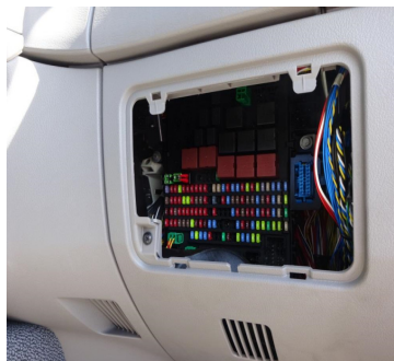
Figure 7-2.2 Inside View - Electrical Junction Box Location
