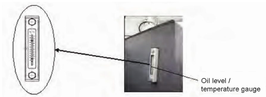
Figure 1-17 Liquid Level Gauge
