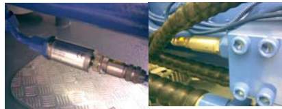
Pressure transducer installation
