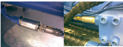
Pressure transducer installation
